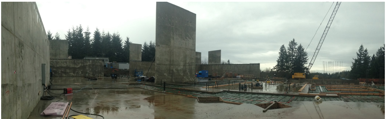
Below: Concrete pour for wall at the west edge of the lap pool.
