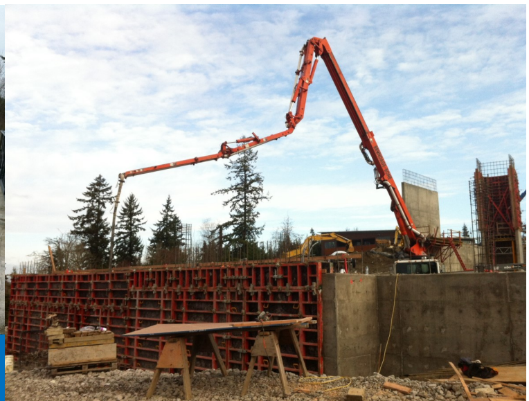
Below: Concrete pour for wall at the west edge of the lap pool.
