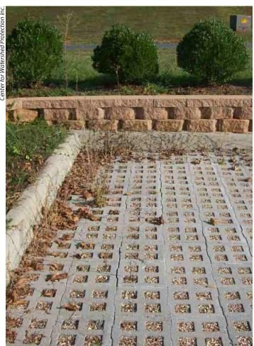
Example of a modular grid pavement parking area in need of maintenance. Leaves and debris pose clogging hazards, and reduce infiltration.
