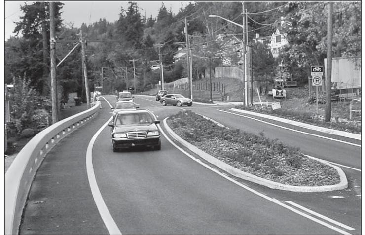
*Looking north along the parkway, the new bikelanes, median strip, and turning lane are visible. In the background, a car makes a left turn onto a side road from the new turning lane. A sidewalk has also been added on east side of the parkway.*
