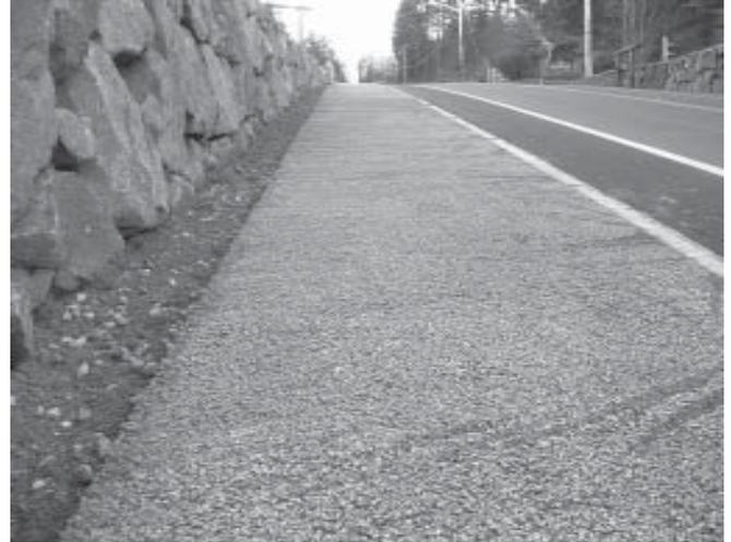
*New porous concrete sidewalk near the intersection of SE 24<sup>th</sup> Street and 239<sup>th</sup> Avenue SE.*
