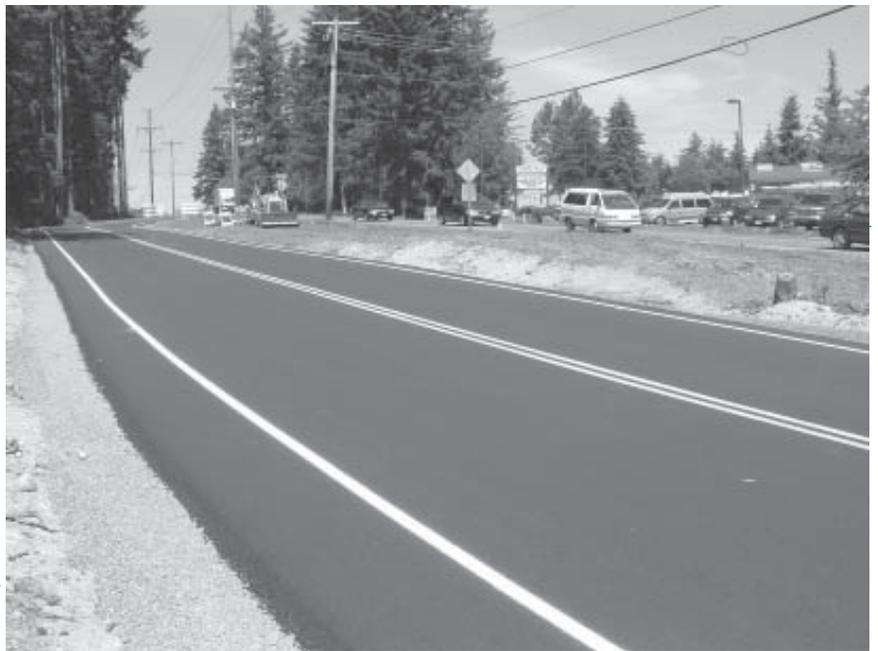
The temporary bypass road along Issaquah-Pine Lake Road is shown shortly before it opened for use earlier this month. The newly paved detour will allow utilities to be relocated under the permanent road in the background.
