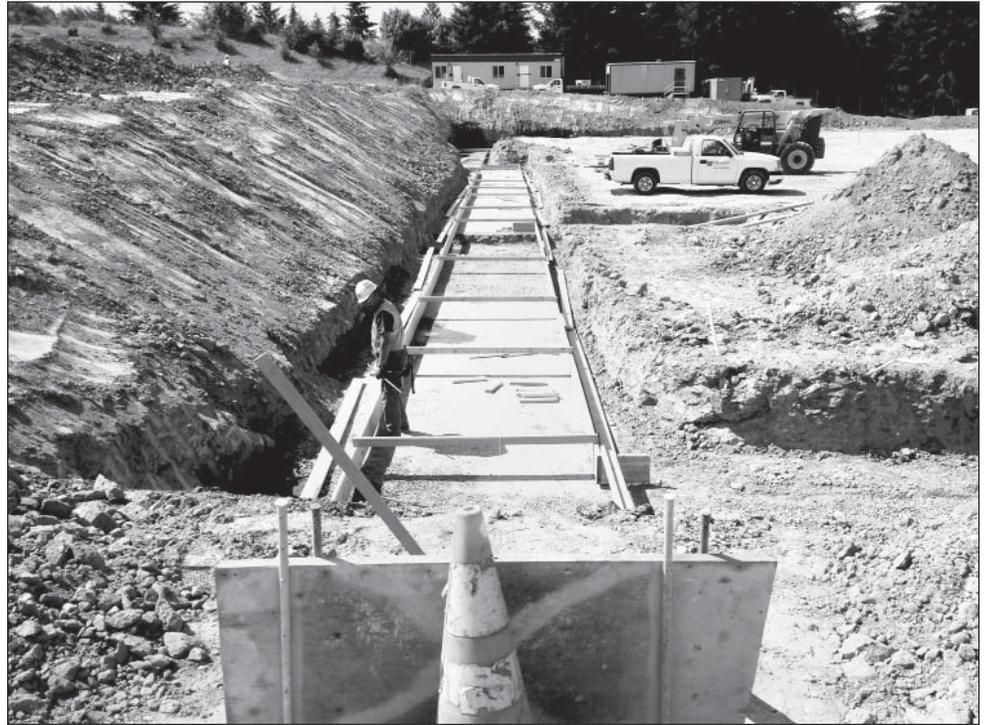
*As grading continues elsewhere on the site, the foundation formwork goes in for the eastern wall of the new, 69,000-square-foot Community & Aquatic Center.*
