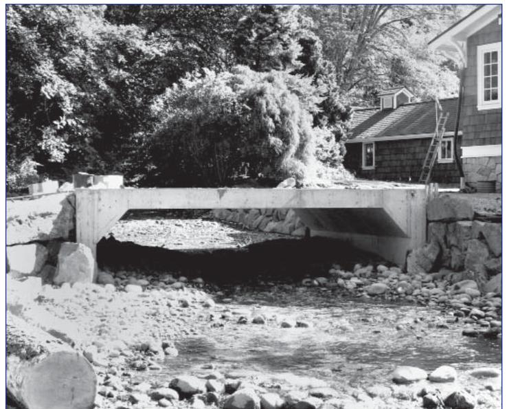
*This is the expansive box culvert that replaced the 18-inch pipe. It was paid for by property owner Wally Pereyra.*
