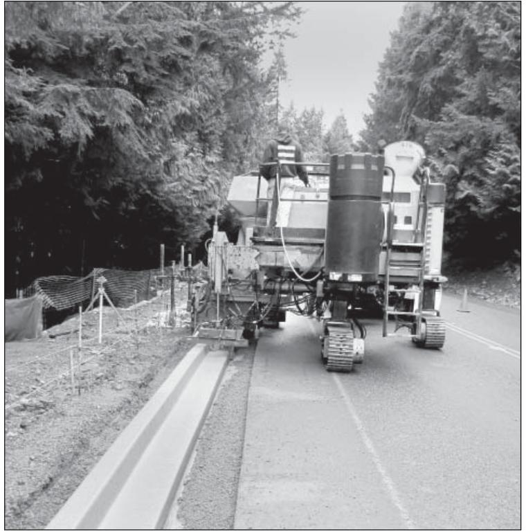
*A curb machine lays down cement concrete along Inglewood Hill Road.*
