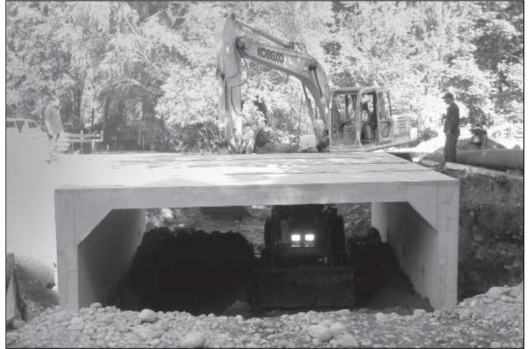
*This is the 20-ton box culvert Wally Pereyra installed to replace the pipe.*
