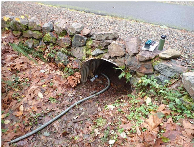
Photo 1 Upper George Davis Creek under driveway culvert near 223 rd PI NE. Note sediment buildup
