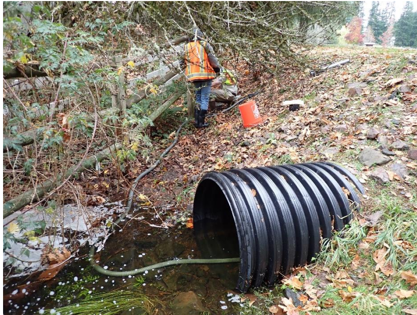
Photo 2 Upper Ebright Creek gauge site at outlet of culvert in Big Rock Park North. Note clean pipe bottom and low velocities upstream of fence
