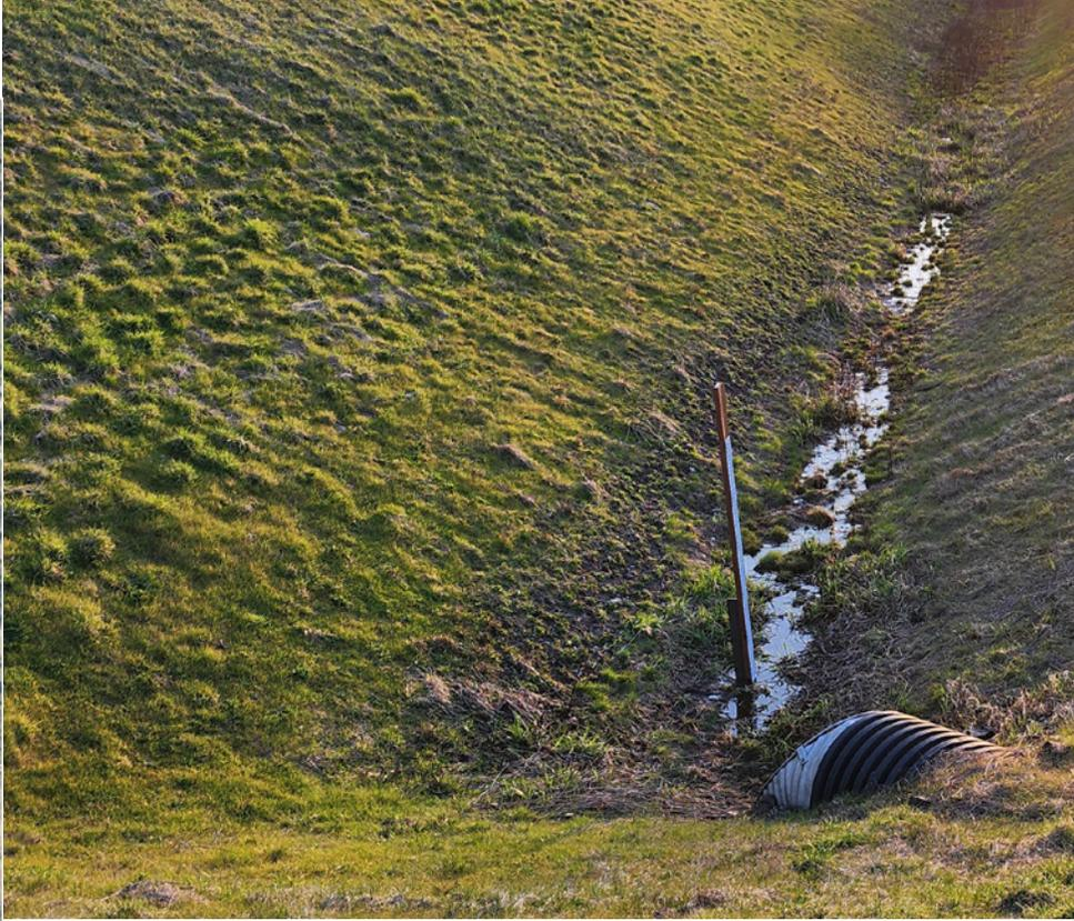
*You may notice new equipment in this photo: these are gauges that allow staff to track how high the pond water levels are and help staff respond and prepare for large rain events.*
