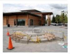
The plaza is prepared for the concrete stair-step base. The structurally engineered base was built in 4 separate concrete pours by Ahmet Baran.
