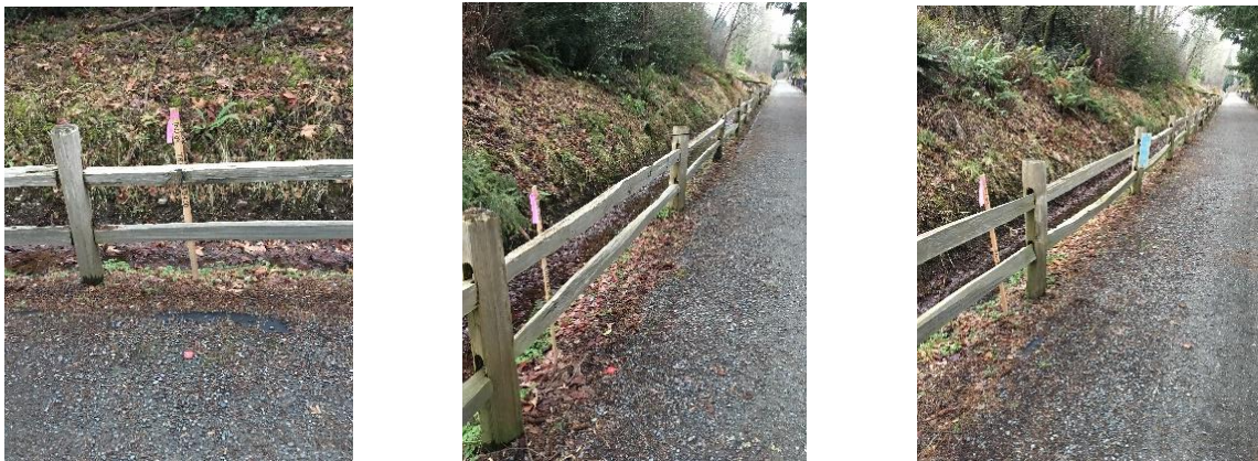
Pictures of sections 375+00 through 376+04 just north of Mint Grove looking south showing that center line of trail is moved east by approx. 6 ft into the area of the ditch and shrubbery.
