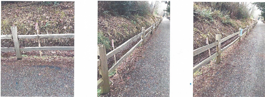
Pictures of sections 375+00 through 376+04 just north of Mint Grove looking south showing that center line of trail is moved east by approx. 6 ft into the area of the ditch and shrubbery.
