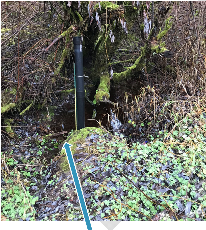
FIGURE 5. HAZEL WOLF CULVERT
