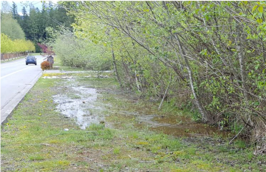
FIGURE 7. FLOODED DITCH ADJACENT TO 248 TH AVE SE.
