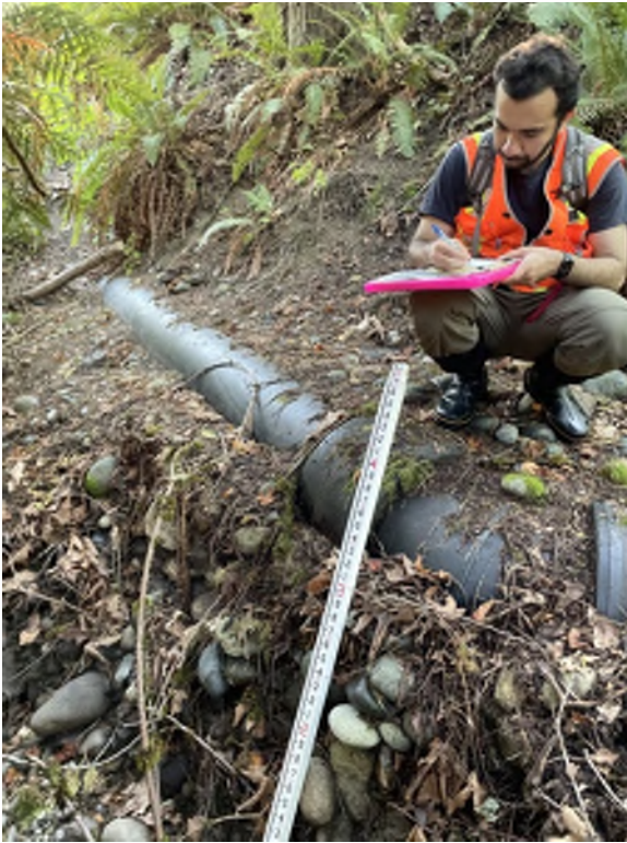
Photo 15. Stormwater outfall pipe and gabion dissipation structure on left side of channel looking upstream. Outfall pipe discharges stormwater from Stormwater Pond D92929 at STA 8400 near 210 th PI SE (September 2023).
