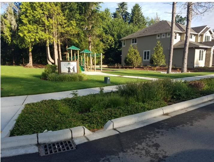
*New developments often incorporate rain gardens or bioretention swales into roadway design to meet stormwater requirements.*
