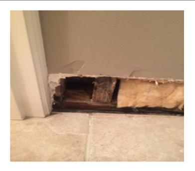
\*Note – The above photo depicts the pathway by which water, forced up through the foundation from hydraulic pressure, runs along the interior walls of the residence.
